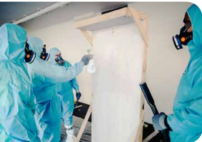
A new suite of training courses, including the Asbestos Worker Program, is part of our long-term investment in the future of the industry.
